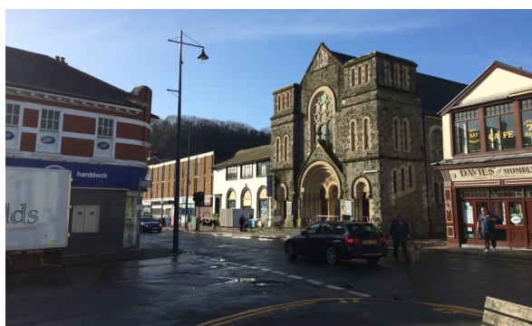
The Dunns with the Methodist Church and commercial unit opposite on Mumbles Road
